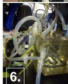
6. Remove the thin overflow-pipe at the T-piece on the storage water heater. Take the thin hose of the mains inlet valve and attach it to the T-piece instead.
